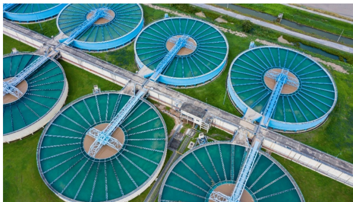
Photo: Ariel view of water treatment plant.jpg
